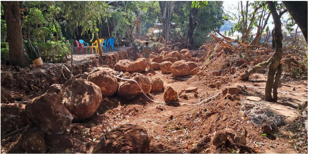
Figure 5: New road under construction (photo by first author, February 16, 2025)
